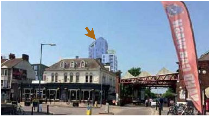
Figure 10 - Hove Gardens viewed from Goldstone Villas
